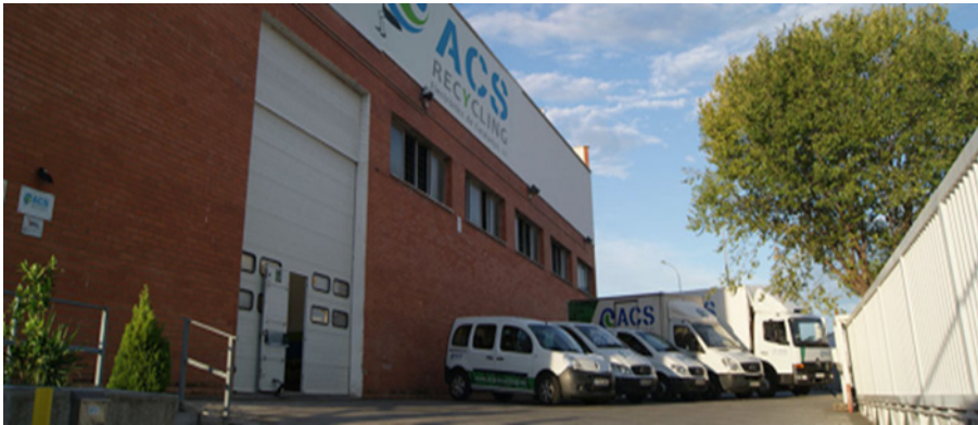
Figure 5: ACS recycling facilities
